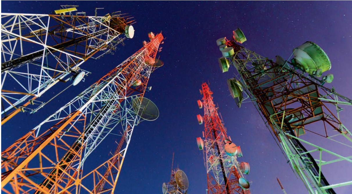
Telecommunication masts with microwave links. Microwave technology can send data from the UK to Germany and back again in less than five milliseconds – a twentieth of the time it takes to blink an eye
